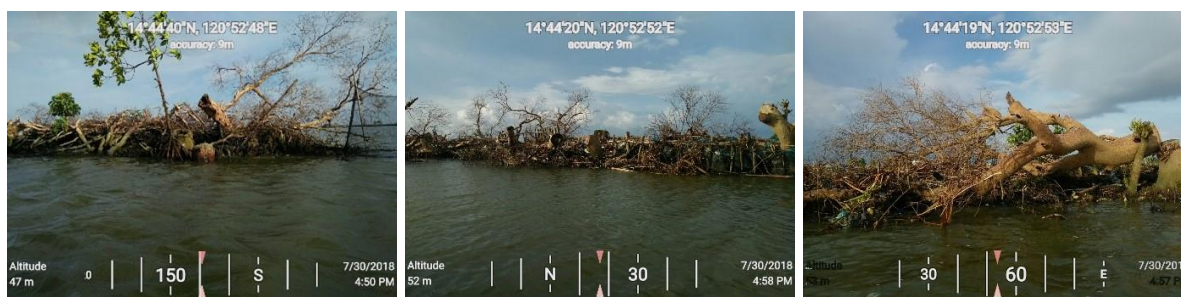
Geotagged photos conducted on a spot visit by local government officials in Bulacan show the destruction of mangrove trees in San Miguel’s airport development area in 2018.
